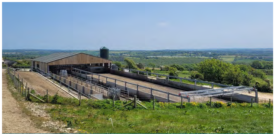
The family has recently completed the installation of a 54-bale Waikato rotary parlour
